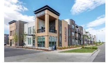
Springs at Peña Station 210 units – Planned 2022
