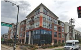
Alta SOBO Station 187 units – 2019
