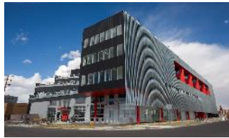
Zeppelin Station 100k SF retail/office – 2018
