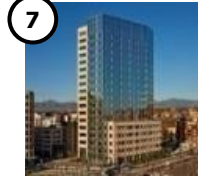
1900 16th STREET (2009) 17 Story Office, Retail & Living Space
