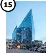
TRIANGLE BUILDING (2015) 11 Story Office, Retail
