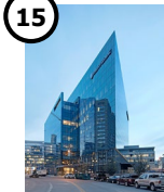
TRIANGLE BUILDING (2015) 11 Story Office, Retail
