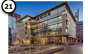
N. WING BUILDING (2013) 5 Story Office, Retail, Restaurants & Parking
