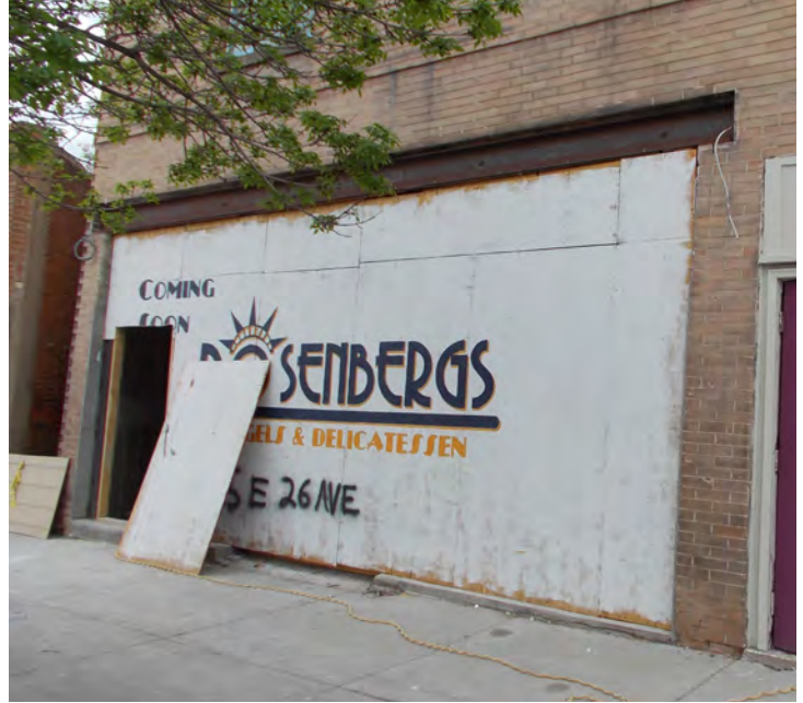
BEFORE - E 26TH AVE FACADE
