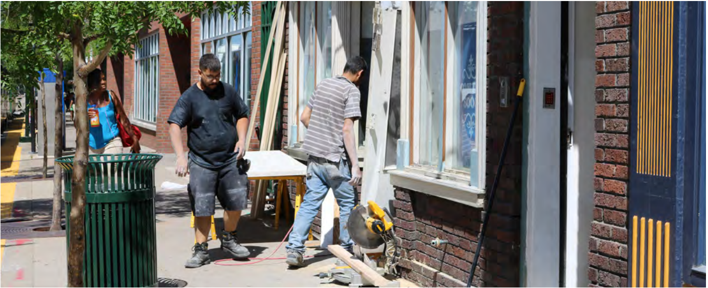
Reuse and rehabilitation work underway on a Main Street Character Building.
