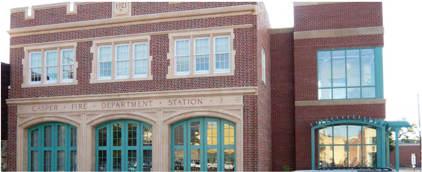
A contemporary addition, on the right, to an historic Fire Station in Casper. The addition features a change in wall plane and similar window and door proportions that complement the original windows and doors. The addition has simplified ornamentation.
