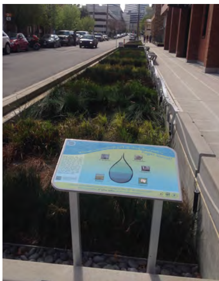
Water quality planters filter pollutants and debris from stormwater runoff, providing a valuable service to the city. To maintain proper functioning, these devices need regular maintenance, especially after a storm event.
