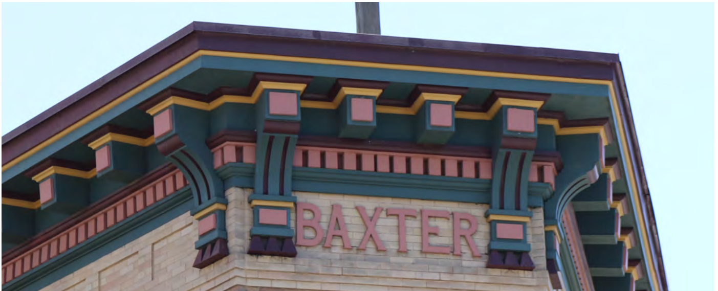
An historic upper story wall sign incorporated into the architecture of the building. The letters are individually pin mounted and are placed between the cornice corbels and sized appropriately in the available space.
