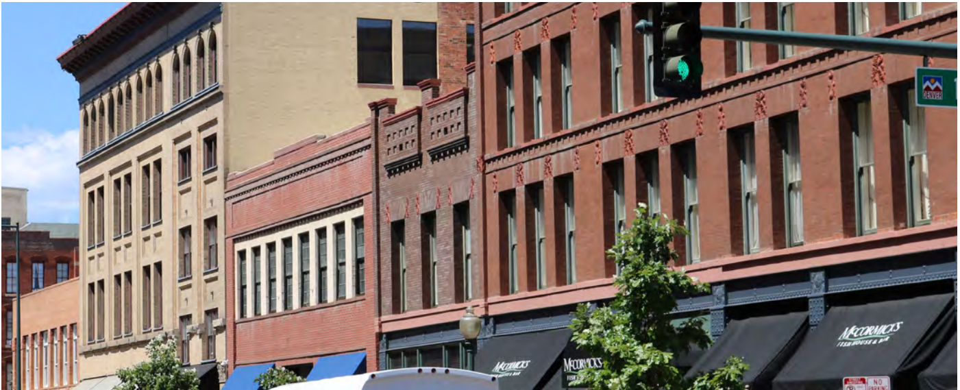
Facade articulation techniques, such as belt and string courses, cornices, storefront piers, a floor-to-floor alignment, used in the image above creates a cohesive street frontage while providing variety along individual building facades.
