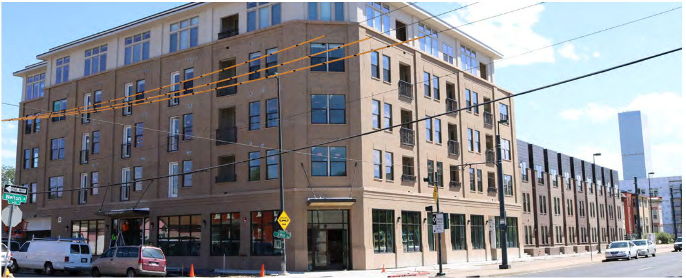
This large infill project that is shown under construction is built at the property line, creating a strong street edge, and maintaining the Character-Defining Features of the cultural district.
