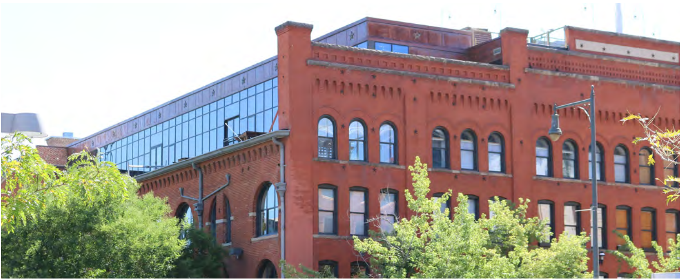
A contemporary addition with a compatible roof form and similar materials.
