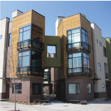
Innovative residential infill development
