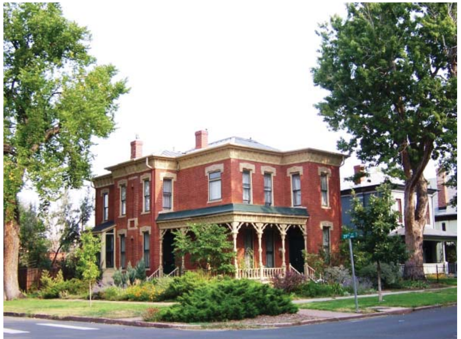
Curtis park has some of the oldest residential structures in Denver, such as this 1880s Italianate-style home
