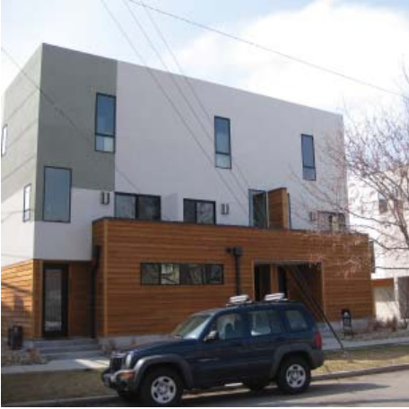
Urban Residential infill in Curtis Park
