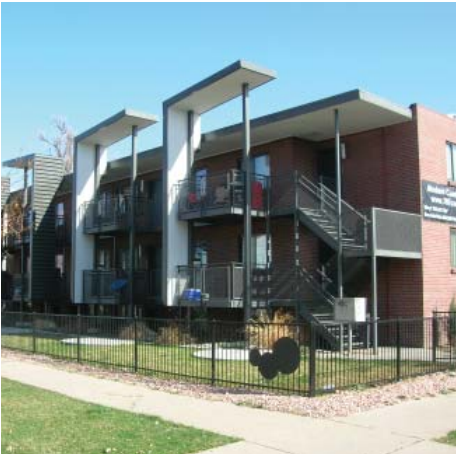
Apartment buildings are being retrofitted into for-sale condominiums
