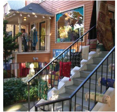
Homes along commercial corridors can be reused as retail storefronts. Homes facing Downing Street could be utilized in a similar manner as these homes in the Nob Hill neighborhood of Portland.
