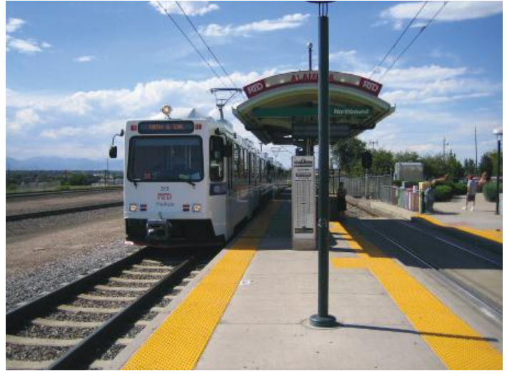
Picture 1.3 Alameda Station Platform Looking North
