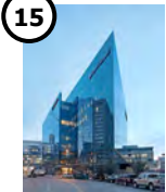
TRIANGLE BUILDING (2015) 11 Story Office, Retail
