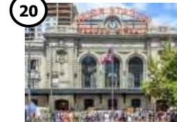
DUS HISTORIC BUILDING (2014) 112 Room Crawford Hotel & Retail
