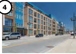
ALTA CITY HOUSE (2015) 5 Story, 281 Apartments
