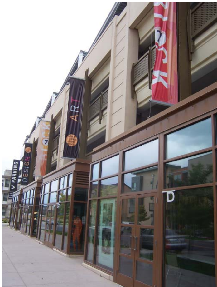
Belmar’s Block 7 Studios and Galleries demonstrates a flexible approach to activating parking structures
