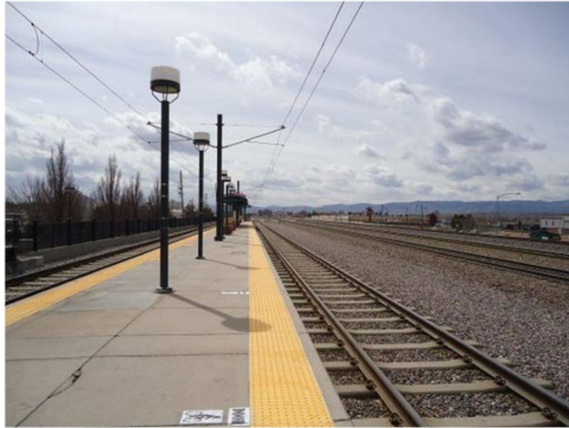
FIGURE 2 EXCLUSIVE ALIGNMENT ADJACENT TO FREIGHT RAIL CORRIDOR
