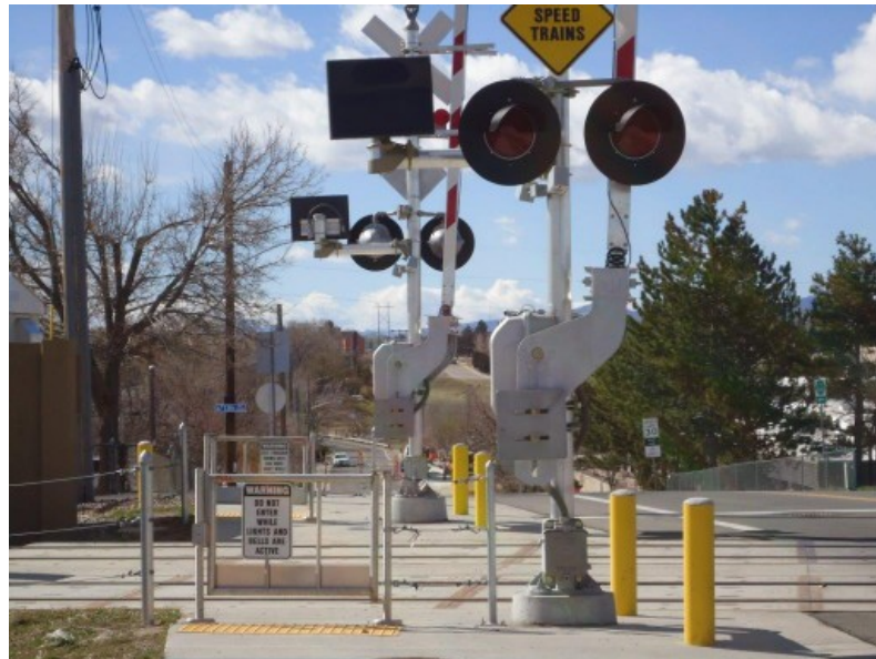
FIGURE 8 - PEDESTRIAN CROSSING WITH SWING GATES
