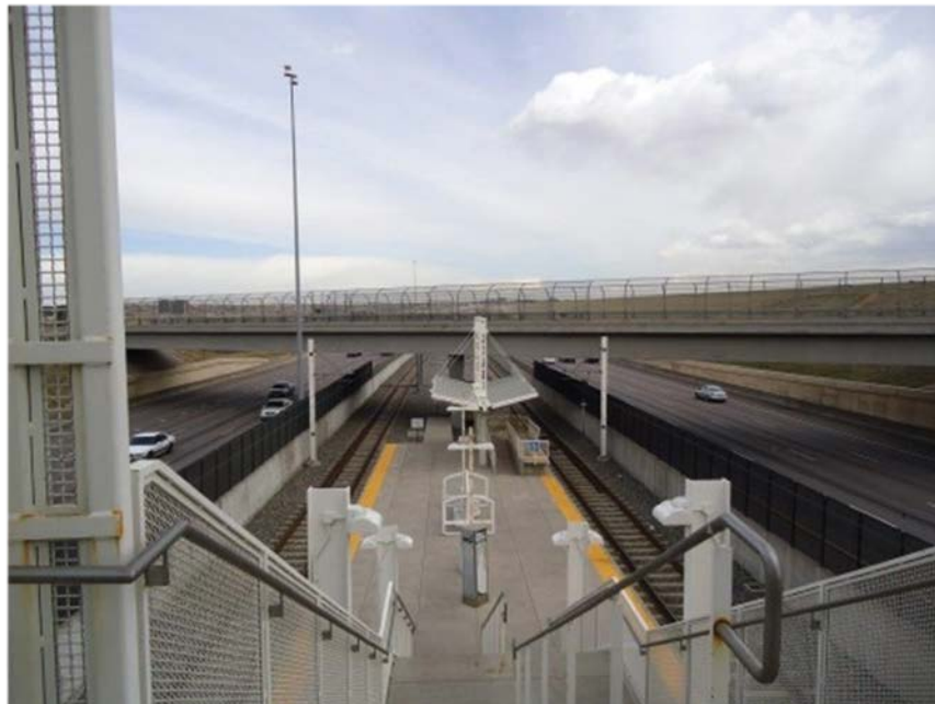
FIGURE 1 – EXCLUSIVE ALIGNMENT IN HIGHWAY MEDIAN
