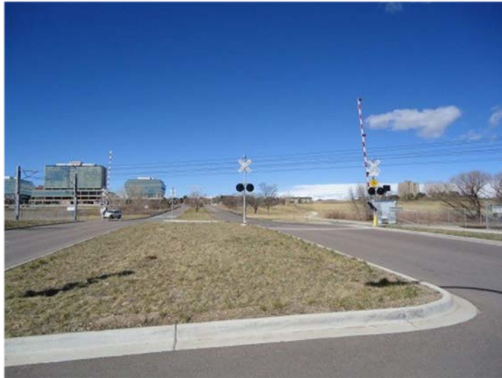
FIGURE 5 – TYPICAL BI-GATES WITH MEDIAN TREATMENT
