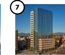
1900 16 th STREET (2009) 17 Story Office, Retail & Living Space
