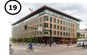
S. WING BUILDING ONE UNION STATION (2014) 5 Story Office, Retail
