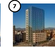
1900 16 th STREET (2009) 17 Story Office, Retail & Living Space
