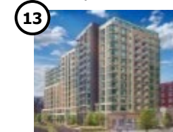
THE PULLMAN (2020) 14 Stories, 3K Retail, 164 Apartments
