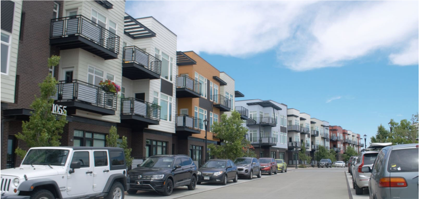
Figure 40: New DELO Apartments east of the BNSF rail line (looking north)
