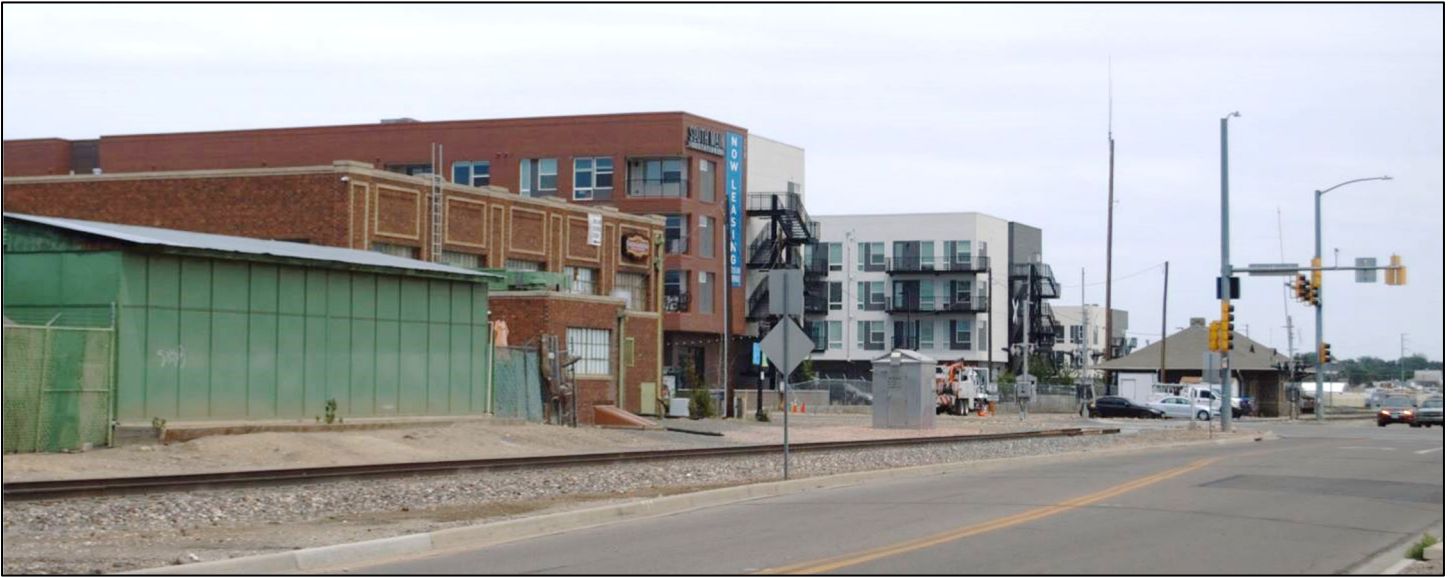
Figure 54: New development east of US 287 (Main Street) in Longmont
