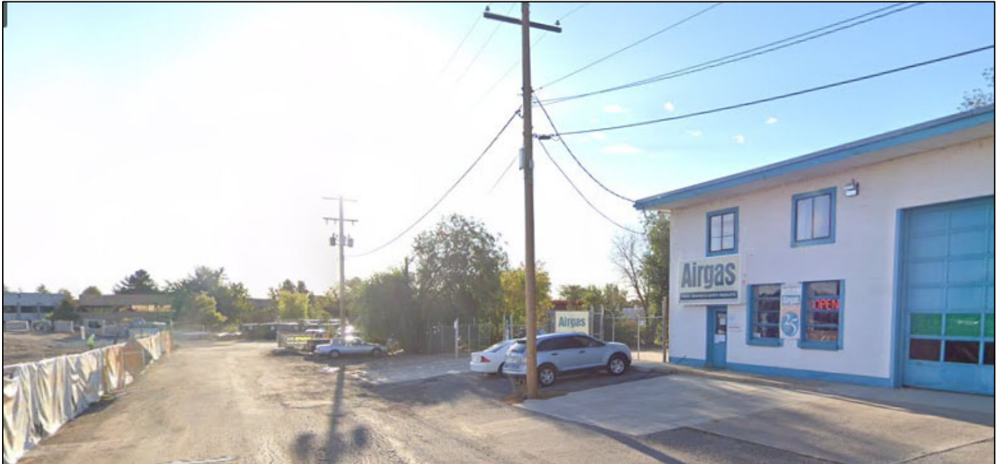
Figure 44: Overhead Utility Lines on Bluff Street Near Proposed Boulder Junction at Depot Square Station
