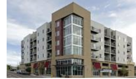
Garden Court at Yale Station 64 affordable units – 2016
