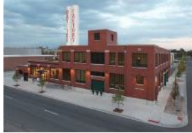
Dry Ice Factory 20k SF office – 2009
