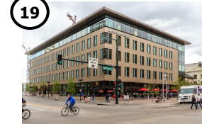
S. WING BUILDING ONE UNION STATION (2014) 5 Story Office, Retail
