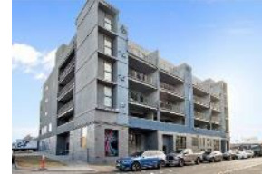
Factory Flats 24 condos – 2018
