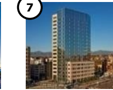
1900 16 th STREET (2009) 17 Story Office, Retail & Living Space
