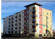
University Station Apartments 60 senior units – 2014
