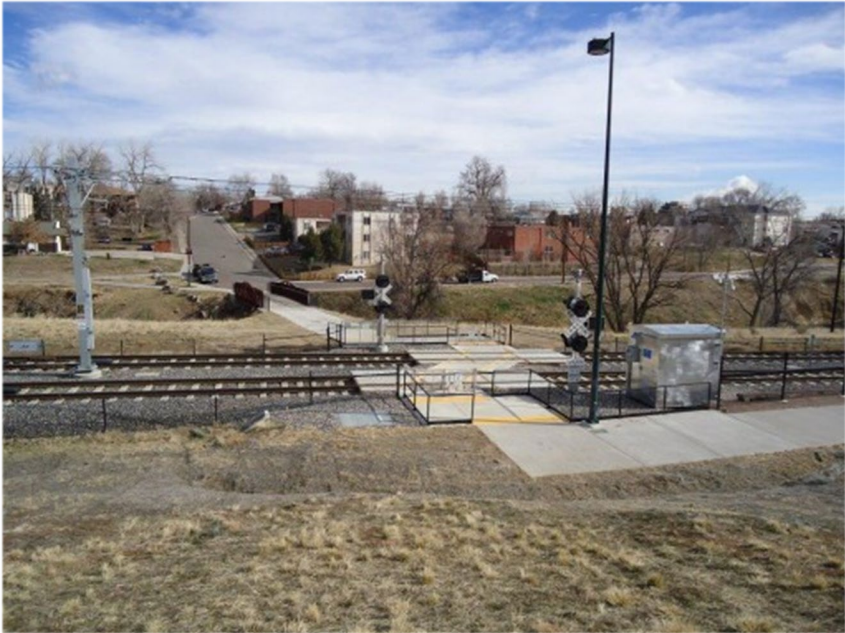
FIGURE 9 - PEDESTRIAN CROSSING WITH Z CROSSINGS
