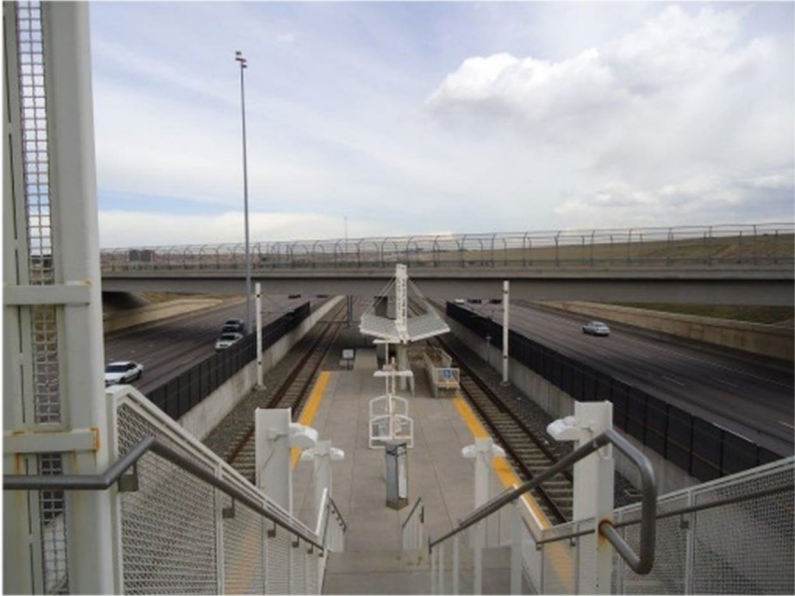
FIGURE 1 – EXCLUSIVE ALIGNMENT IN HIGHWAY MEDIAN
