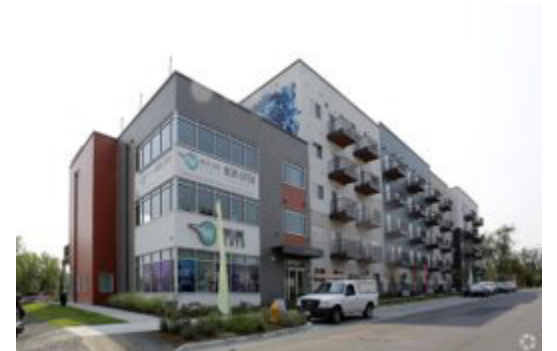
West Line Flats Lamar Station
