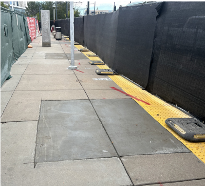
Colfax at Auraria Station Concrete Repairs
