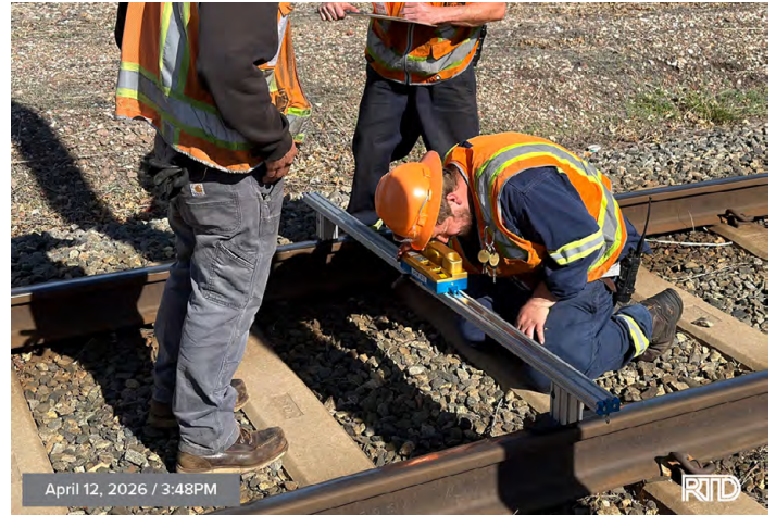
Verifying Wire Height and Alignment Ball Arena | April 12 3:48 PM
