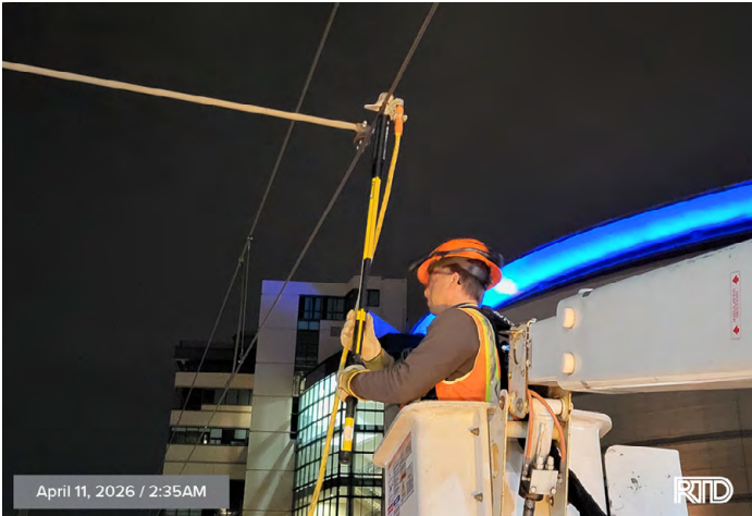
Grounding the Overhead Wire Ball Arena | April 11, 2:35 AM
