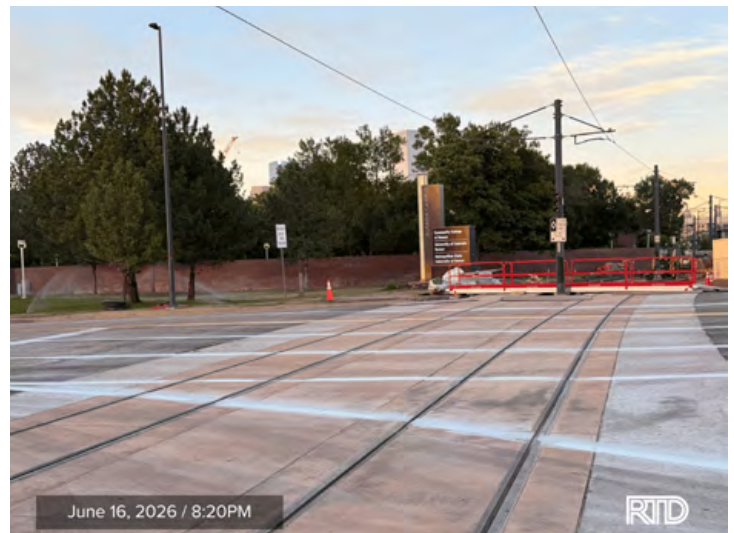
Reconstructed Rail Crossing Seventh Street Crossing | June 16, 8:20 PM
