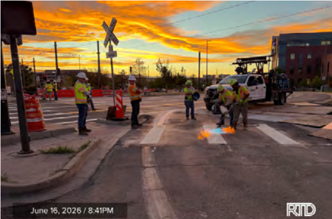
1 | Installing Crosswalk Striping Seventh Street Crossing | June 16, 8:41 PM
