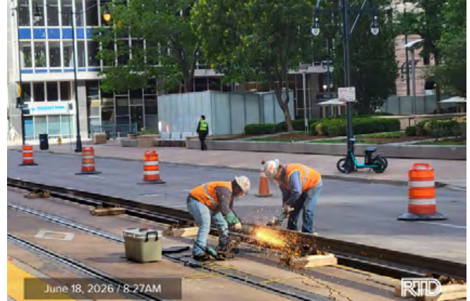
2 | Rail Grinding Downtown Loop | June 18, 8:27 AM
