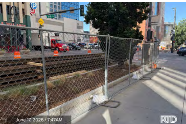
Pedestrian Safety Fences Downtown Loop | June 17, 7:47 AM
