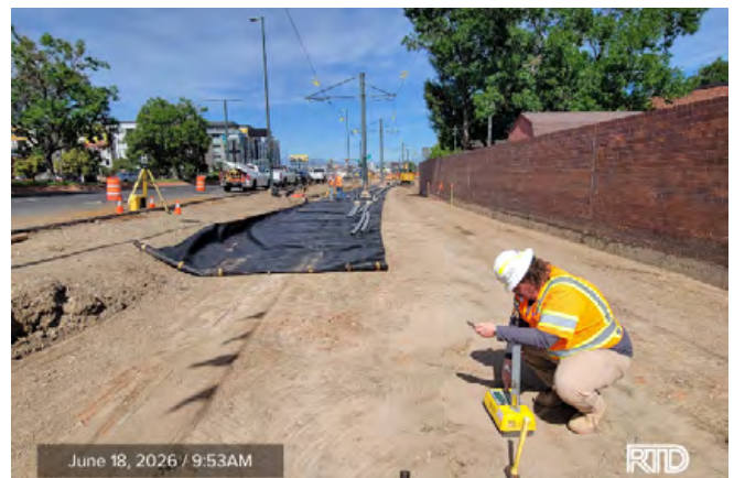
Soil Compaction Test Seventh Street Crossing | June 18, 9:53 AM
