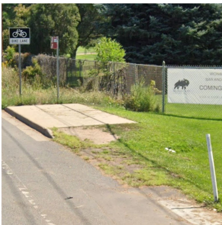
Figure 3-33: Lawn Obstructing Path of Travel at 5700 Block Arapahoe Ave in Boulder (12237)
