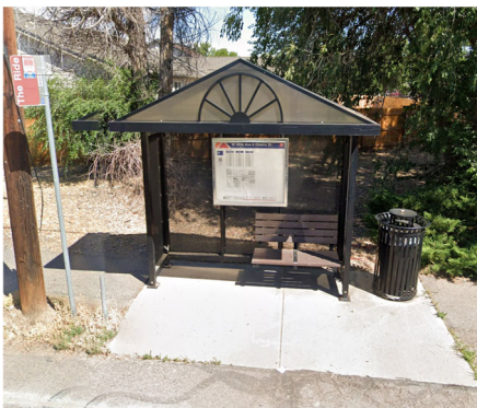
Figure 3-46: Permanent Shelter at W 38th Ave & Parfet St in Wheat Ridge (11033)
