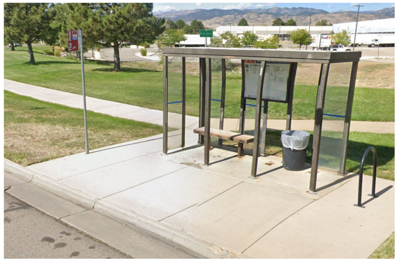
Figure 3-39: Unverified Shelter Clearance Limitation at Spine Rd & Williams Fork Trail in Boulder (16631)
