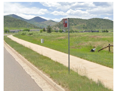
Figure 3-11: Missing Pad at W Coal Mine Ave & S Ward St in Unincorporated Jefferson County (24575)
