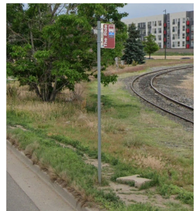
Figure 3-35: Debris Obstructing Path of Travel at W Oxford Ave & Natches Ct in Sheridan (25032)
