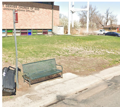
Figure 3-10: Pad Size Limitation at Monaco Pkwy & MLK Blvd in Denver (15554)
