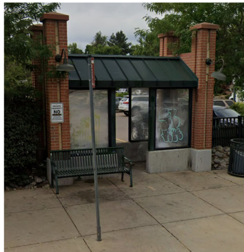
Figure 3-57: Shelter Lighting at 6th Ave & Corona St in Denver (11454)
