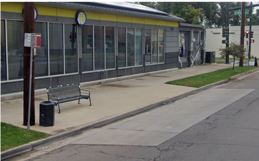
Figure 3-67: Bus pad at W 38 th Ave & Wolff St in Denver (11061)
