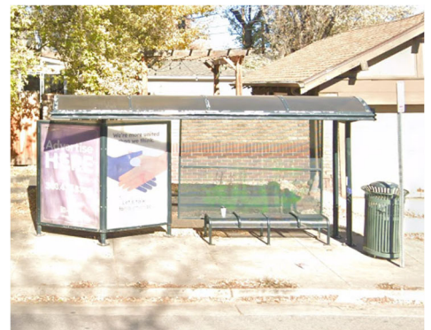
Figure 3-48: Deficient Shelter at 8th Ave & Colorado Blvd in Denver (11830)
