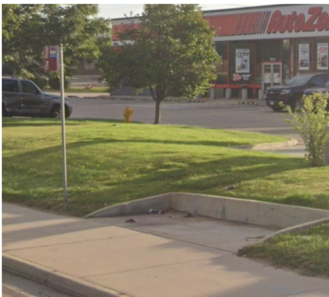
Figure 3-20: Pad Slope Limitation (Not Field Verified) at Federal Blvd & W 95th Ave in Westminster (13775)
