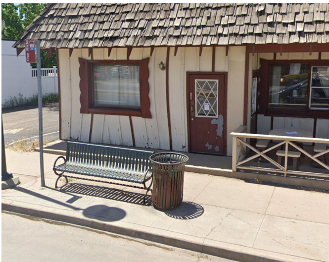
Figure 3-43: Sufficient Bench at S Broadway & W Union Ave in Englewood (12607)
