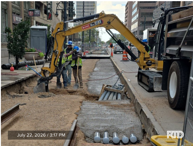
1 | Duct Bank Trench Excavation Downtown Loop Area | July 22, 3:17 PM
