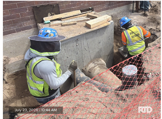
2 | Drainage Inlet Backfill and Compaction Colfax Avenue Alignment | July 23, 10:44 AM
