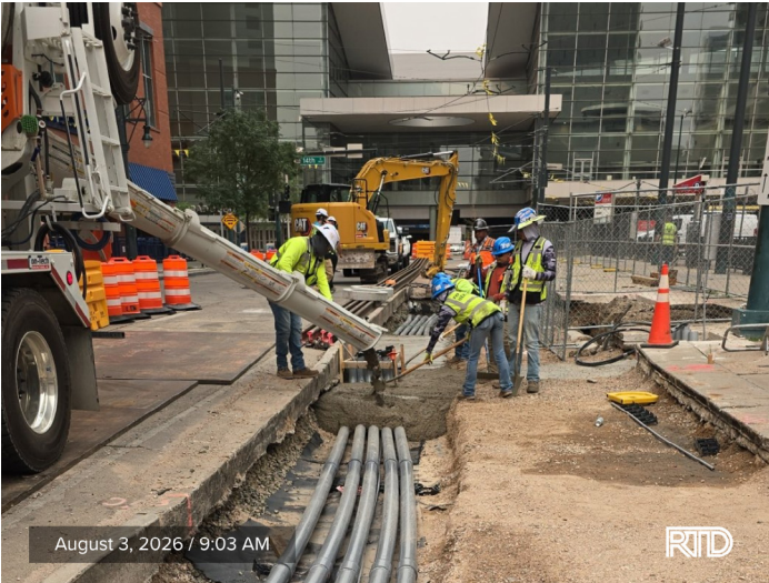
1 | Self-Compacting Material Pour Downtown Loop Area | August 3, 9:03 AM
