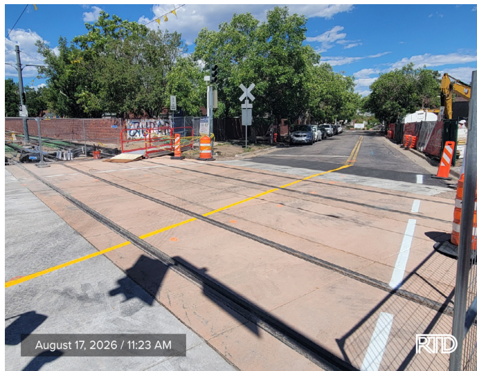
Completed Ninth Street Crossing Colfax Avenue Alignment | August 17, 11:23 AM
