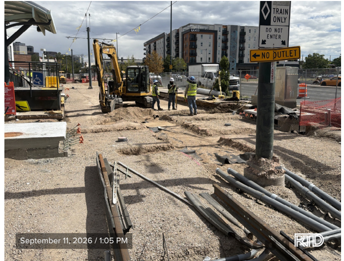
Excavation for Underground Duct Banks Downtown Loop Area | September 11, 1:05 PM
